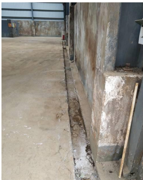
危废仓库防泄漏沟
